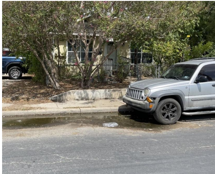
Figure 3: Example of standing water due to service line leak.
