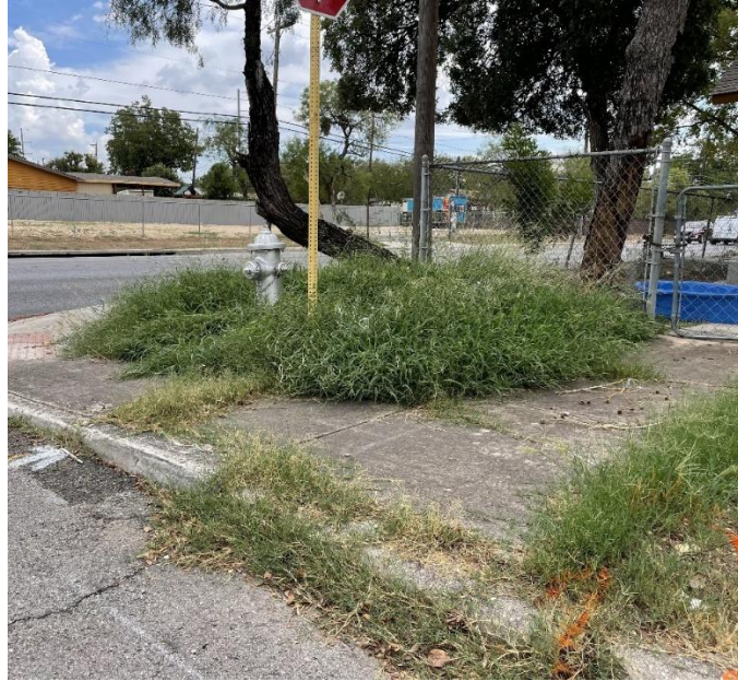
Figure 2: Example of fire hydrant leaking at the seat for an extended period.
